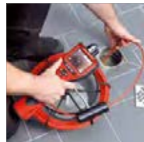
Inspection of floor drains
