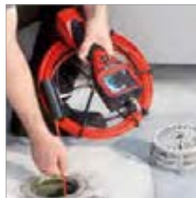
Inspection of rain downpipes
